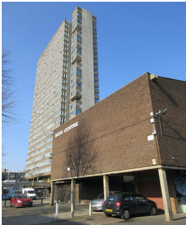
Photo 2.1: Maydew House and the Bede Centre
